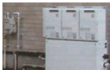
■ Hot water circulation system
